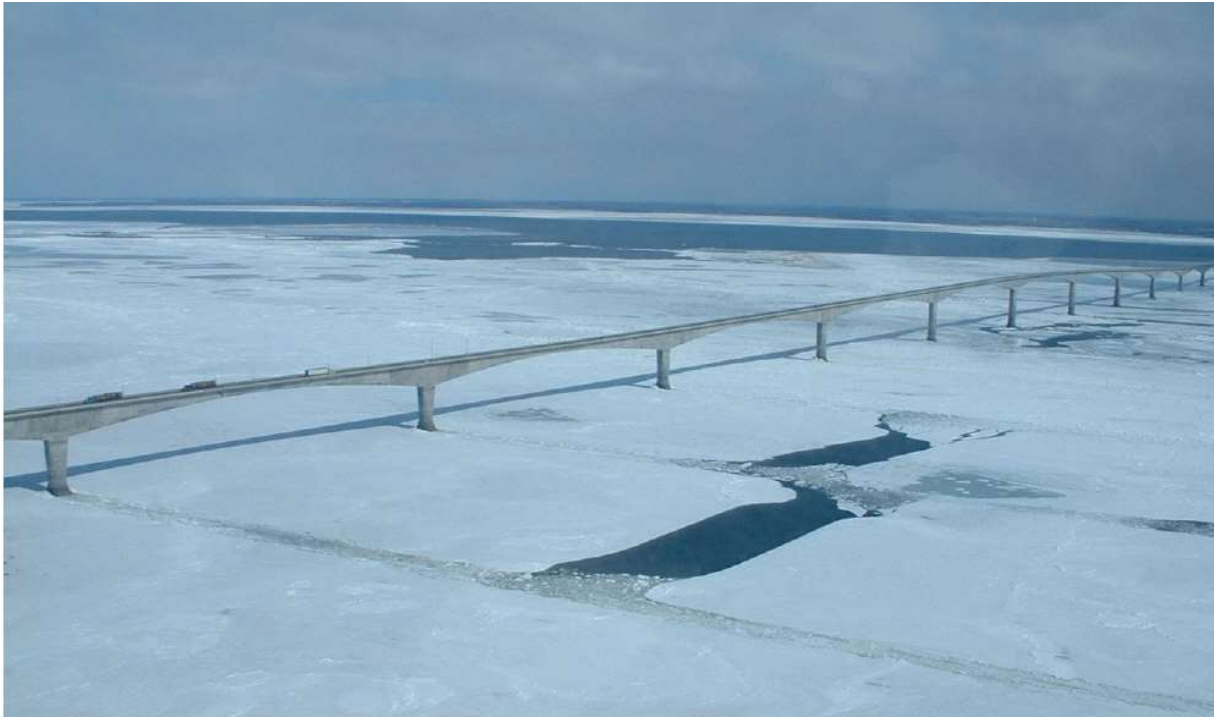
Figure 3. The Confederation Bridge. Government of Canada image.
