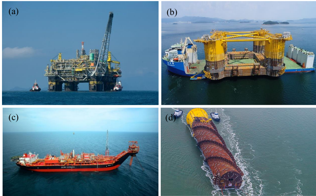
Figure 2-1. Different types of floating structures. (a) Petrobras P-51 Semi-submersible Platform in Brazil (Wikipedia), (b) Shell Appomattox TLP Hull in Gulf of Mexico (Courtesy of COSCO Shipping), (c), Armada Kraken Harsh Environment FPSO in North Sea (Courtesy of Bumi Armada) (d) Gulfstar One Spar in Gulf of Mexico (Courtesy of Williams Partners)
