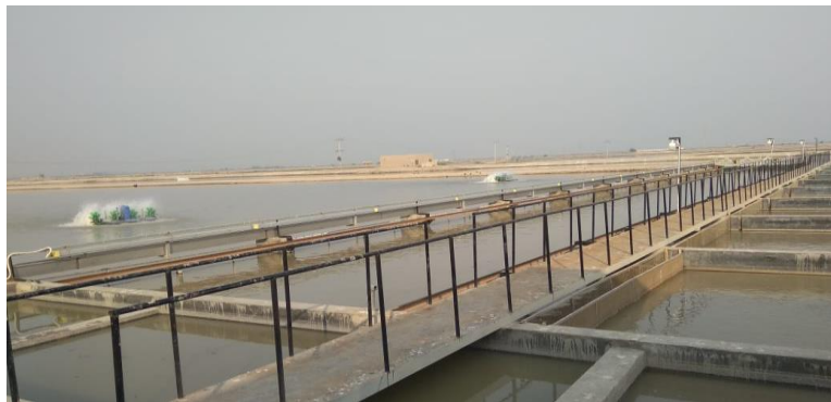
Figure 31. Nursery ponds and aeration blower in operation at the site
