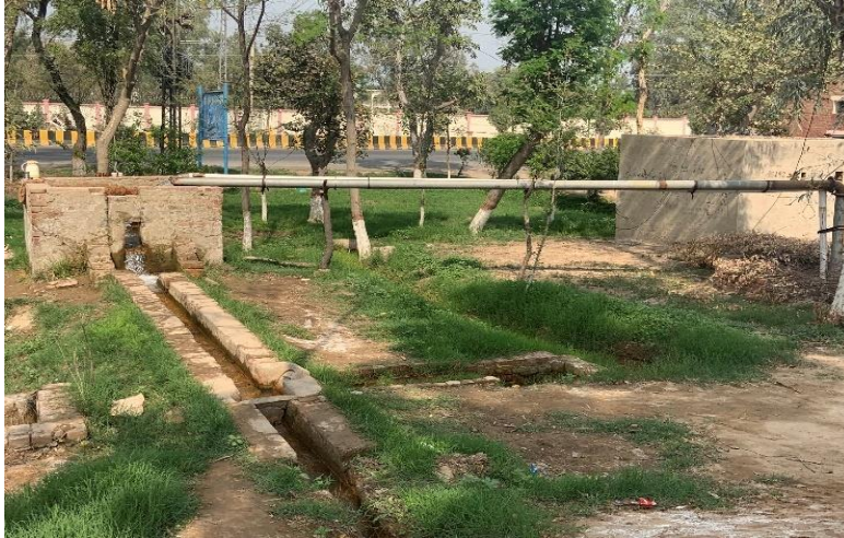
Figure 30. The water pumping system of the fish farm
