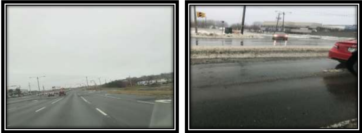
Figure 2.2: Abrasive loss related rutting on Kenmount and Columbus Rd, St. John's
