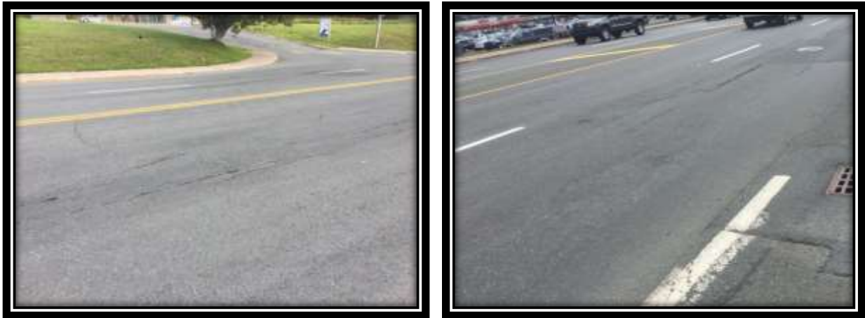
Figure 2.4: Micro-cracking and raveling of new binder mix in different city streets in St. John's.
