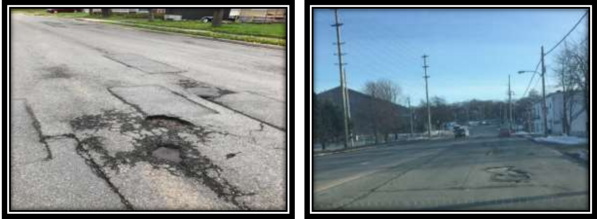
Figure 2.3: Moisture induced damage pothole and delamination in different streets of St. John's
