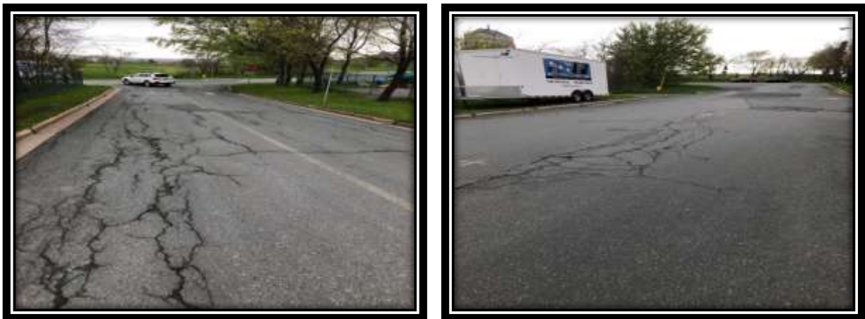
Figure 2.5: Representative illustrations on cracking in different city streets in St. John's.
