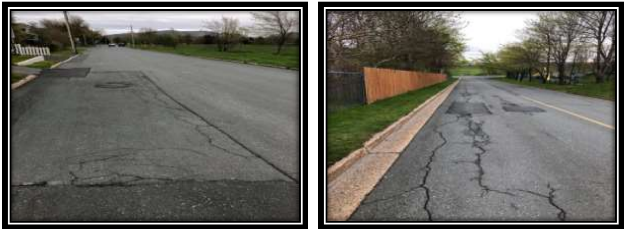
Figure 2.6: Representative illustrations on patching in different city streets in St. John's.
