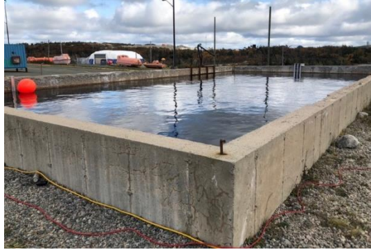
Figure 3-2. Outdoor tank at the Offshore Safety and Survival Center of Memorial University's Marine Institute.
