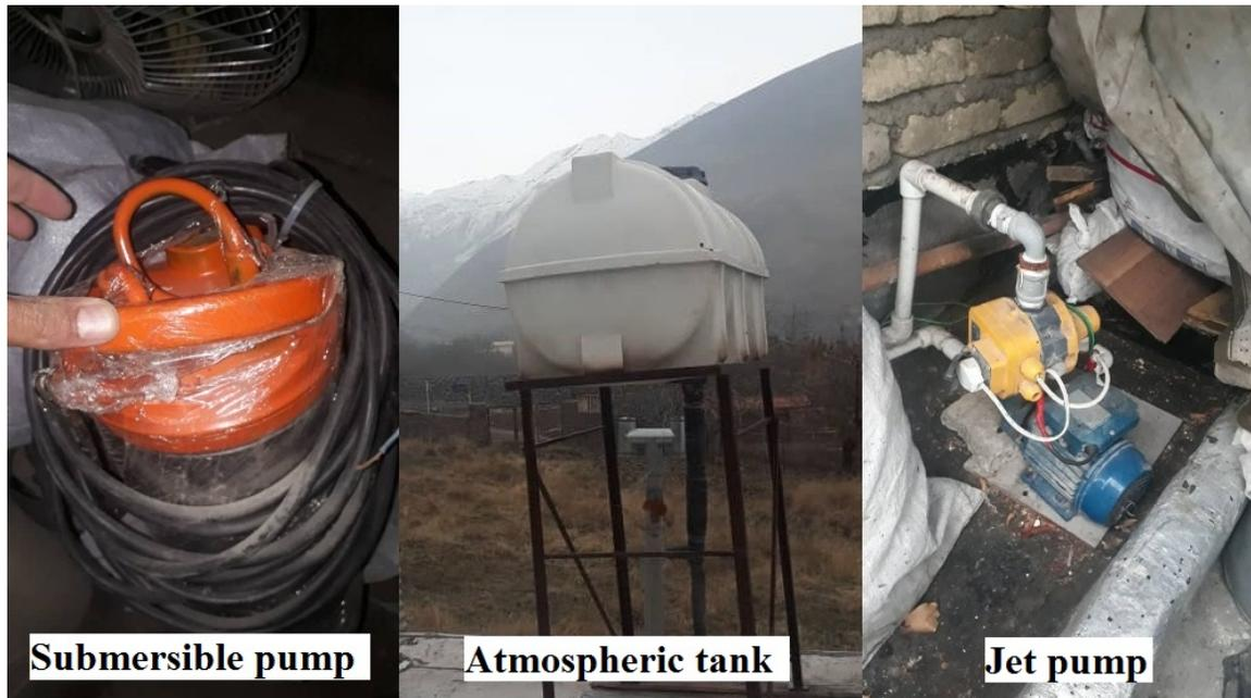
Figure 3.2. Well water system elements in the house
