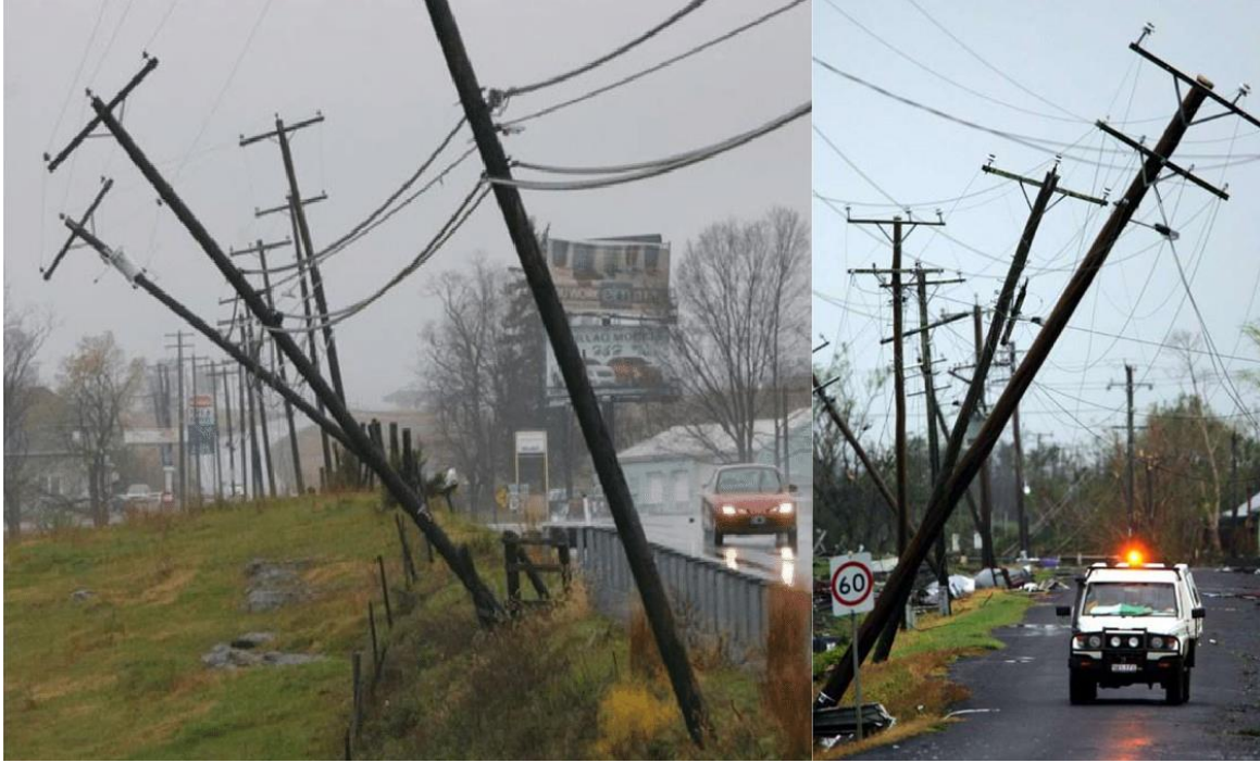
Figure 1.1: Electricity pole failure [4]
