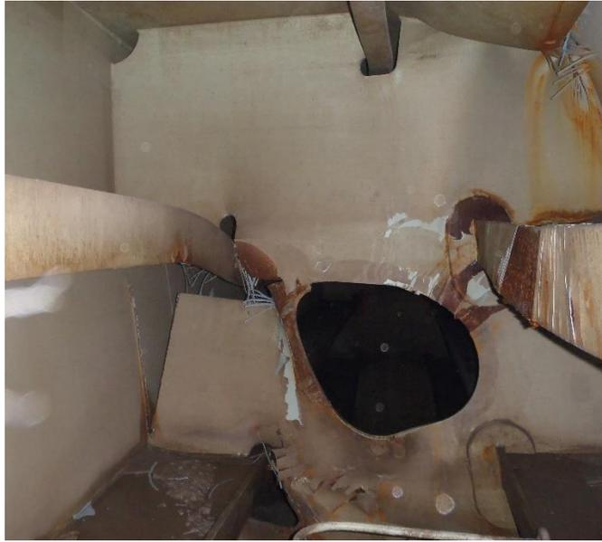
Figure 7-3 Double side structure of a container vessel after collision (taken by the author)
