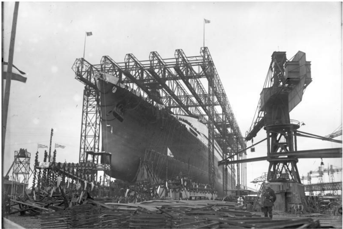
Figure 2-3 - Bremen under construction showing its bulbous bow design [16]
