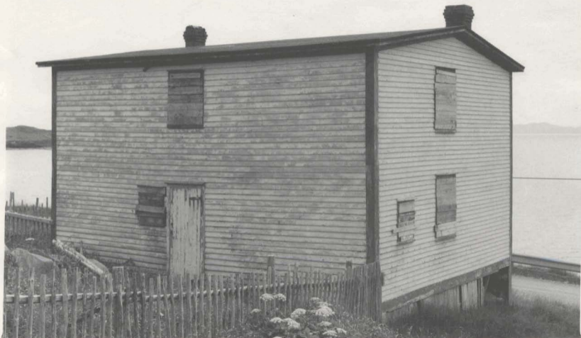
Plate 21 Fourth Generation Two-Storey House, English Harbour, ca. 1915 (Rear View)
