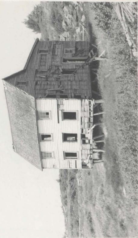
Plate 12 Balloon Framing, near Trinity.
