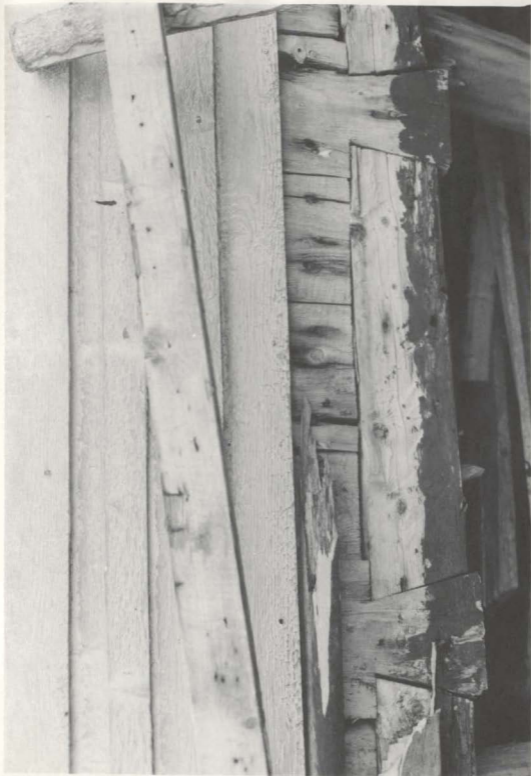
Plate 7 Base of External Studded Wall, Old Bonaventure
