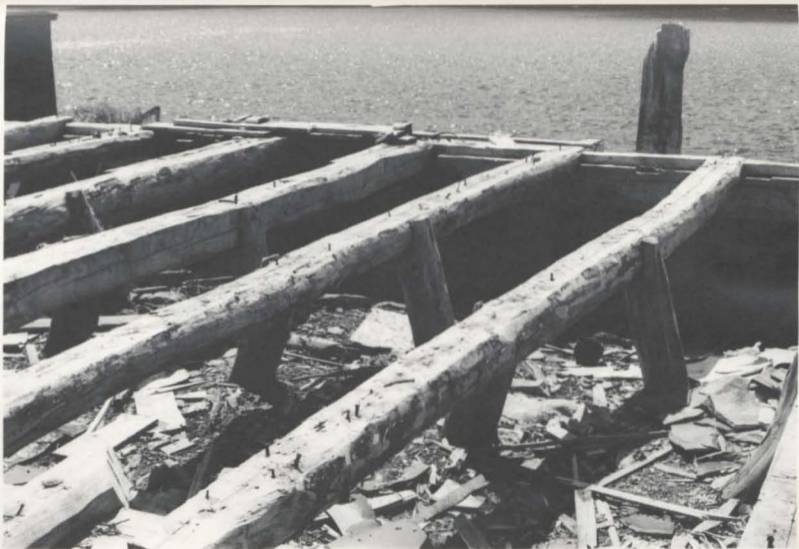
Plate 14 Foundation of Third Generation House, English Harbour.
