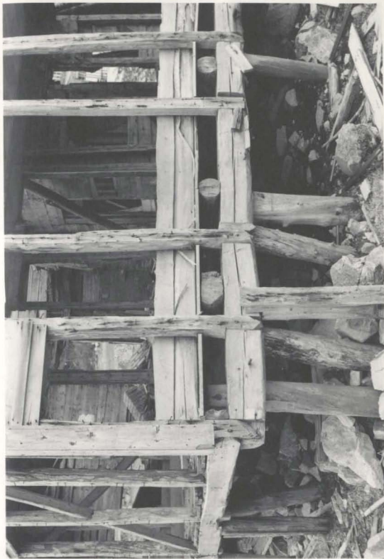
Plate 13 Wall Framing, English Harbour.
