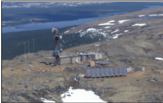
Figure 1: Remote Telecommunications Facility
