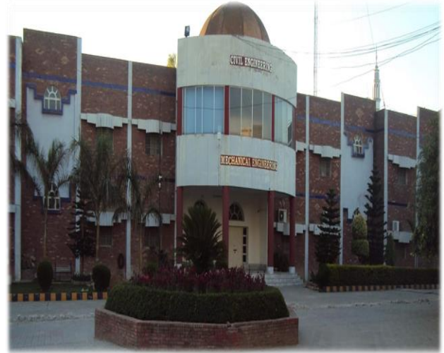
Figure 3 . Front view of the proposed university building.
