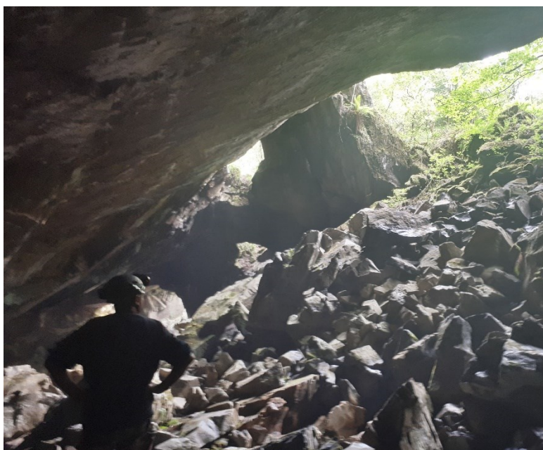
Figure 13: A chamber of Pen-y-Fridd which has been “worked home” to the surface. A dangerously narrow pillar can be seen in the background, and large amounts of rubble from roof collapses are in the foreground.
