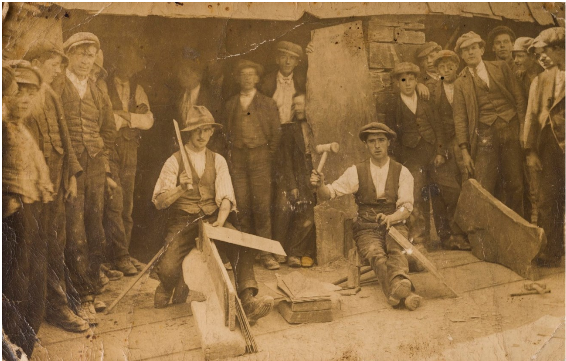
Figure 7: Quarrymen splitting slate and hand-trimming at a trafel outside of the gwaliau at Penrhyn Quarry (Amgueddfa Cymru/National Museum Wales).
