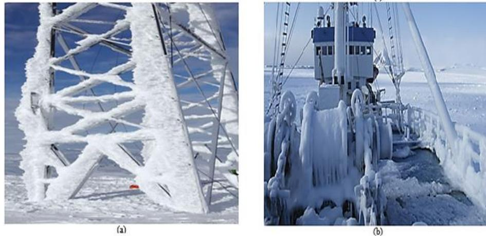
**Fig. 1.1** Ice accretion (a) atmospheric (Hållén, 2015) and (b) sea spray (Ice Sight).
