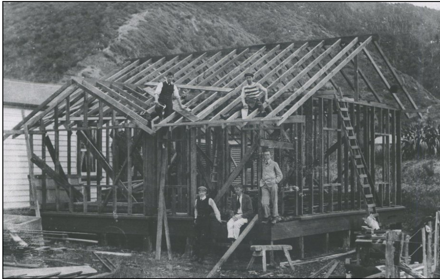
Figure 4-25. A team of carpenters putting together a house at Muritai near Wellington in the early twentieth century (Hocken: 2028_01_002A).
