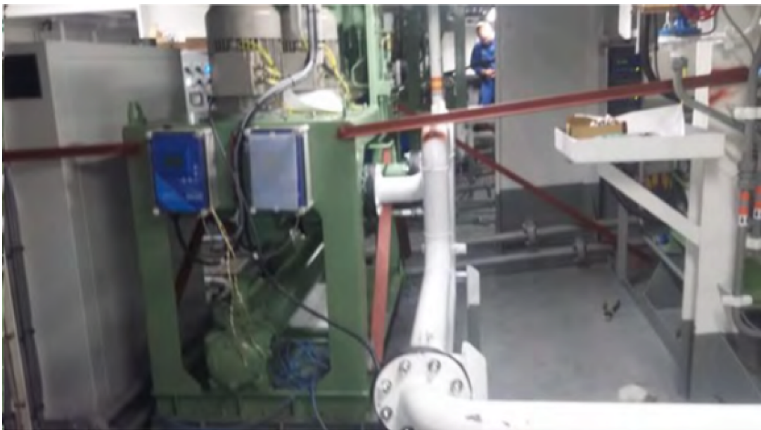
Figure 4: Stiffened electrical oil lube pumps using steel supports (red beams attached to the frame of the green pump and the vessel walls) taken from the Damen Shipyards Report presented to DTW on June 10, 2016 (DTW, 2016c: 667)
