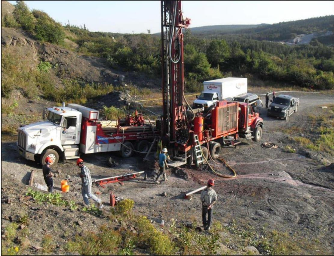
**Figure 42. The field drilling site showing the pVARD tool (left), the PDC drill bit (center) and the SensorSub (right). [48].**
