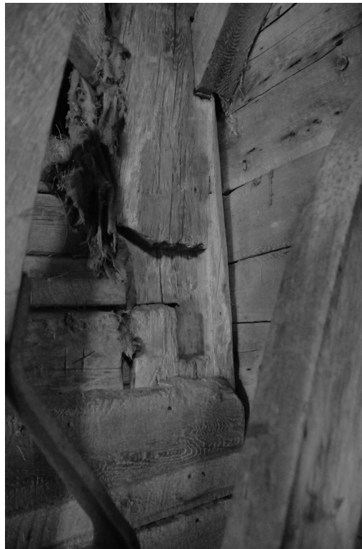
Figure 80. James Fisher barn, Fisher's Mills. Notch pattern to facilitate the placement and removal of the horizontal rail that secures a floor's double doors. Was there once a rear set of double doors in the earliest part of the barn? Is this a recycled post from an earlier structure? When was the brace, visible above, that extends from the post added? Photo by author.
