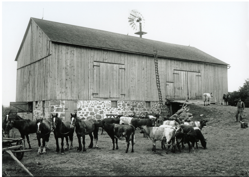
Figure 58. Basement barn in St. Marys, Ontario. Wood and earthen ramp to floor is visible. Circa 1902-06. CI 922. Photograph courtesy of St. Marys Museum and R. Lorne Eedy Archives, St. Marys, Ontario.
