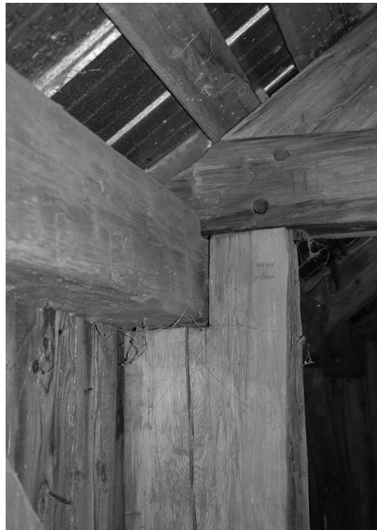
Figure 34. Left: "Flared post" Phase I English barn bent assembly. Note that the flare is exaggerated in the illustration for visual effect. In actuality, St. Mary's barn posts have a less predominate flare. Drawing by Brittany Roberts and labeled by the author. Right: Phase I "flared post" bent assembly in
