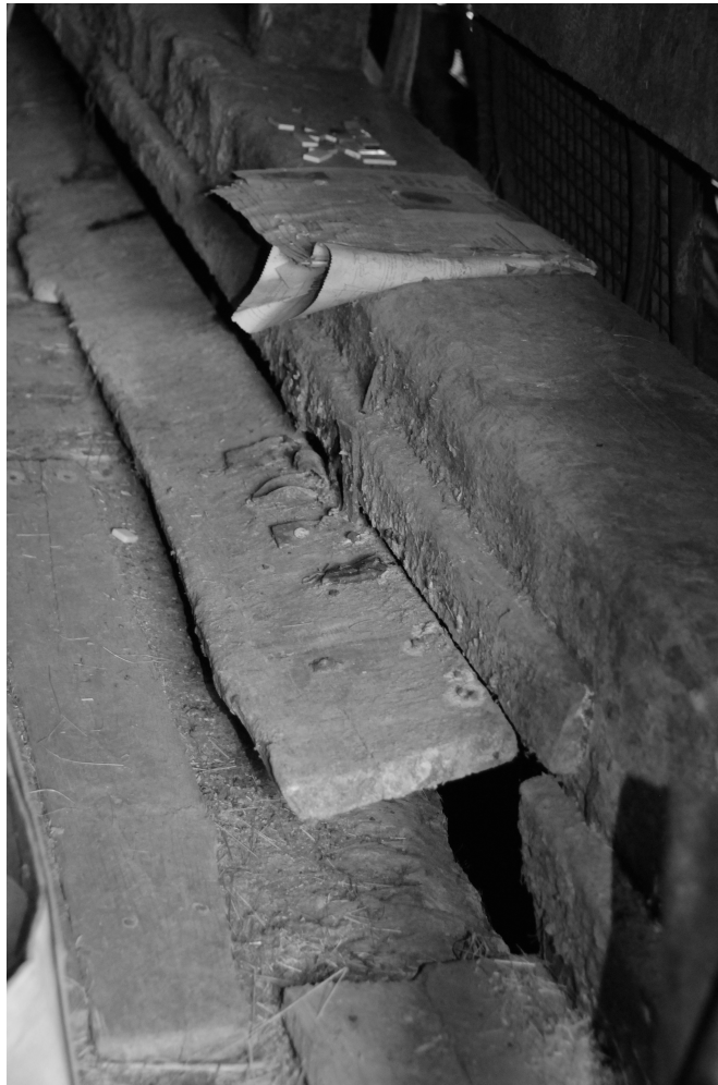
Figure 106. Manure floor hatch, James Fisher barn, Fisher’s Mills. Photo by author.
