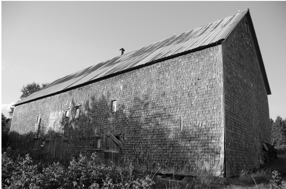
Figure 68. Rear view of George Fisher barn, Fisher's Mills. The large doors of the manure cellar are visible to the left. A vent is at the ridge of the barn to vent the cellar, hay mow, and byre. A small stabling area with door and window is also visible; the use of partial cellar stabling is found only in the later nineteenth-century reformed barns, which will be discussed below. Photo by author.
