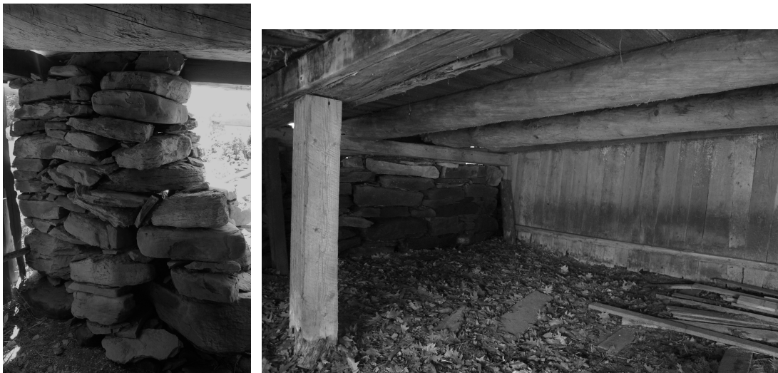
Figure 47. Left: Fieldstone pier supporting the S corner of the Cruickshank barn. Right: Retainer wall of fieldstone against bank, supporting the NW sill. Note also the in-the-round floor joists and the vertical board partition protecting the sunken hay mow from the dirt of the cellar. Photos by author.
