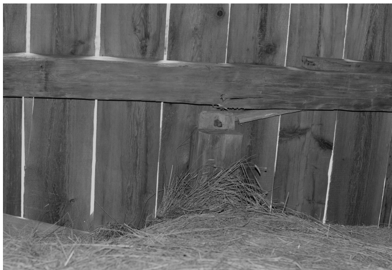
Figure 87. Failure of the central post in the SW gable end bent of the Cruickshank English barn. View taken at loft level. Photo by author.
