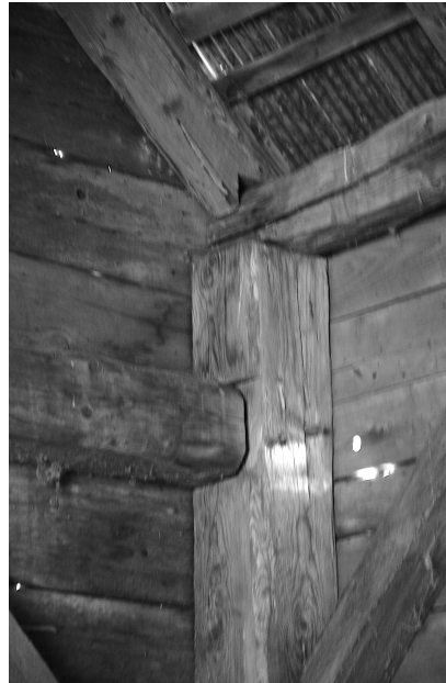
Figure 92. Left: The “straight post with dropped tie-beam” bent assembly. Drawing by Brittany Roberts. Right: “Straight post with dropped tie-beam” bent assembly in the George Fisher barn, Fisher’s Mills. Photo by author.
