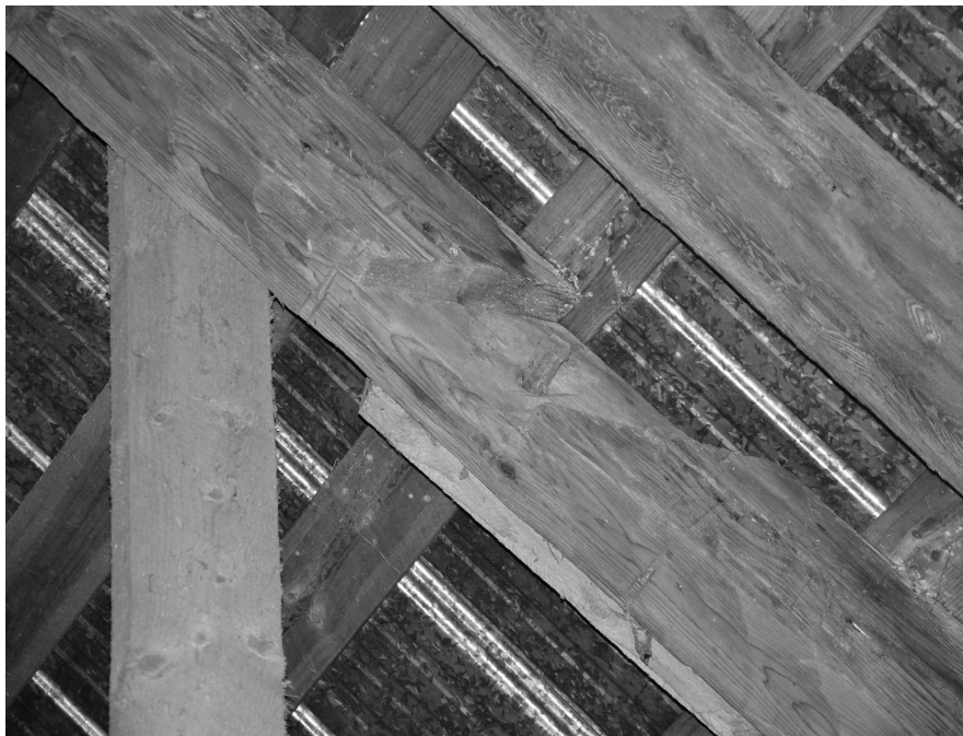
Figure 31. Mortise and peg for a lap joint to connect the now removed collar beam to a gable end rafter, Cumminger barn. The removed collar beam and the two closely spaced rafters shown in this image indicate that the barn was extended at a later date. Photo by author.
