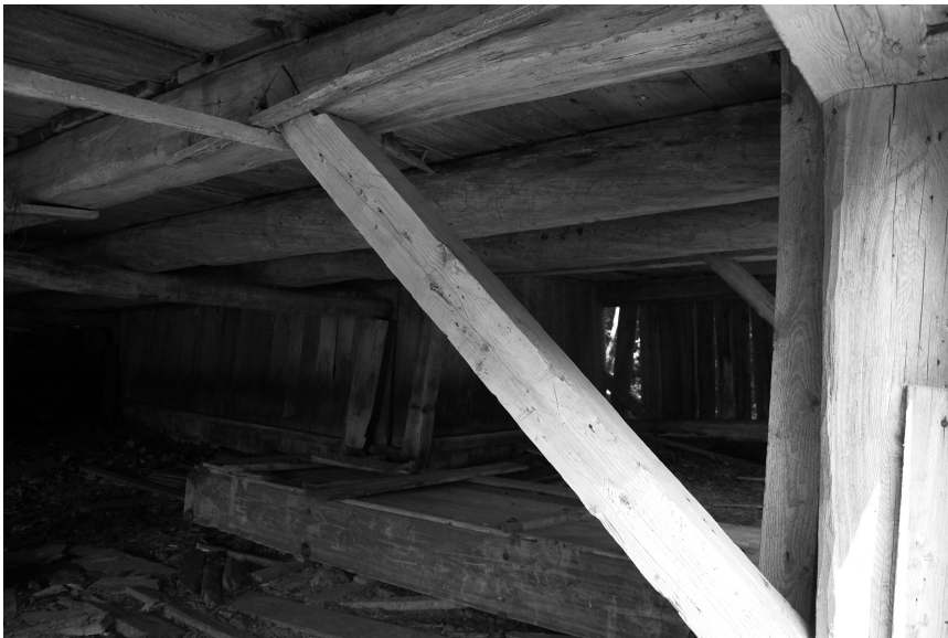
Figure 49. Bracing extending from post into cellar of Cruickshank barn. Note the half-dovetail joint in a squared joist (versus in-the-round). The use of bracing shows that builders were concerned about minimizing barn slide in the side-hill design. Sliding has been an on-going problem for owners trying to preserve their barns. Photo by author.
