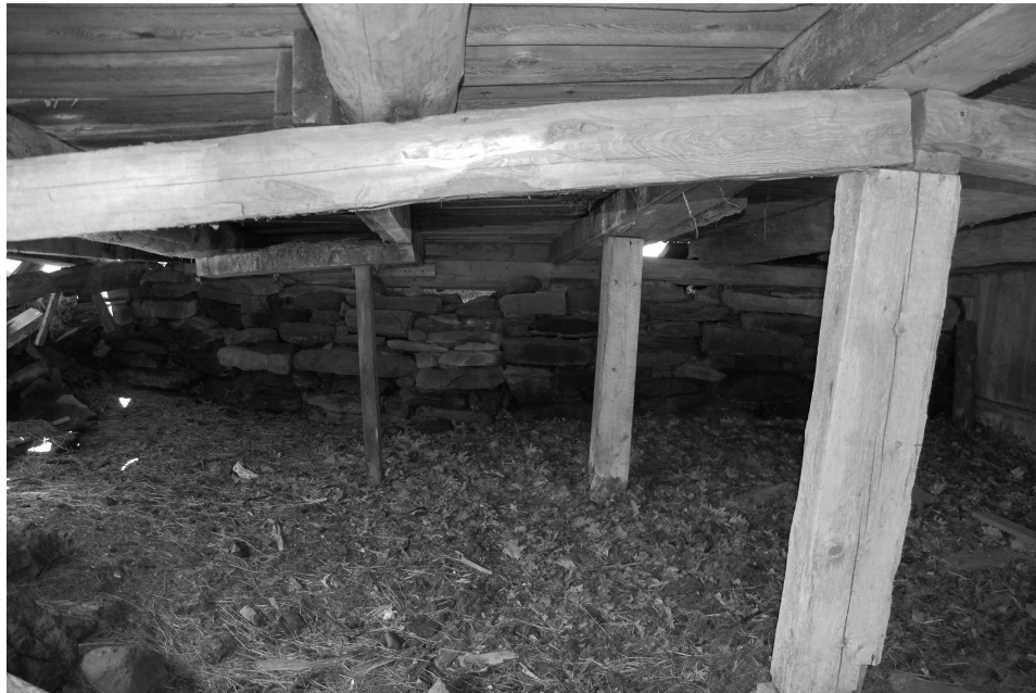
Figure 45. Post supports under the Cruickshank barn. Photo by author.
