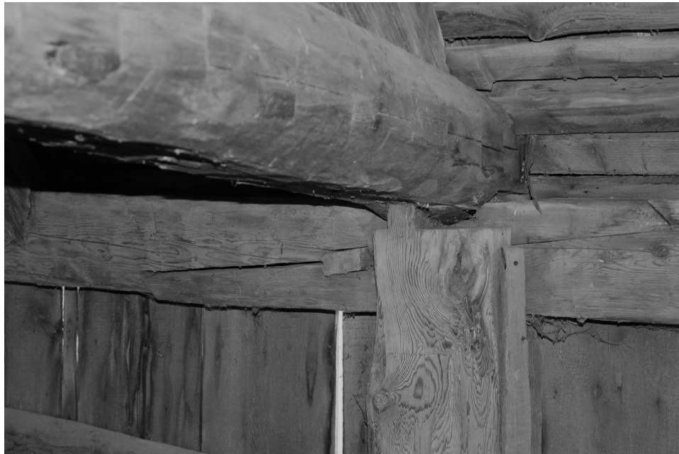
Figure 32. Scarf joint on the wall plate of the Phase II John Henry Jordan barn, Newtown. The tenon of the post is also visible. Photo by author.
