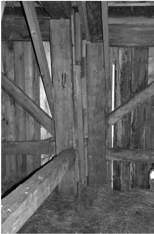
Figure 83. How extension was facilitated in the Cumminger English barn. Left: Looking SE, the end bent of the original English barn is to the left, while to the right is the partial bent of the first part of the extension. Later plank support bracing is visible. Right: Looking NW, the end bent of the original English barn is to the right, while the partial bent of the extension is to the left. The difference between the full and partial bent is clearly visible here—the bent to the left has no tie beam (the hewn rafter sits directly on the wall plate) and no brace extends into the center of the mow from the post. Photos by author.
