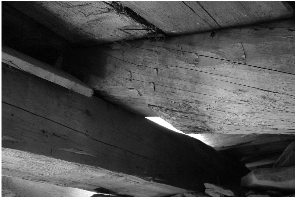
Figure 44. Tapered end of the floor joist of Cruickshank barn, sitting on sill. Photo by author.
