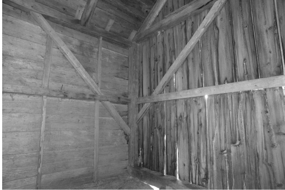
Figure 110. The Cruickshank barn, Caledonia. To the right is the original vertical board sheathing of the gable end of the barn. To the left, the vertical board sheathing, with studs, probably applied when the barn was extended. The boards on this wall are covered with wood shingles. Photo by author.
