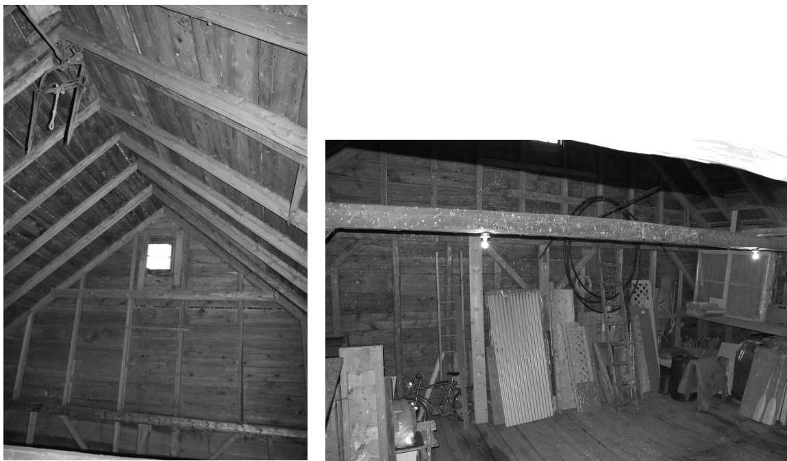
Figure 96. Studded framing in the Cruickshank barn, East River St. Mary's (Left). Studded framing in the Lower Ross barn, Waternish (Right). Photos by author.
