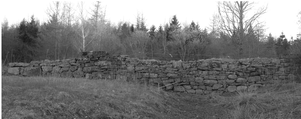
Figure 105. Typical stone retaining wall from the manure cellar of the demolished Erwin Cameron barn, East River St. Mary’s. Photo by author.
