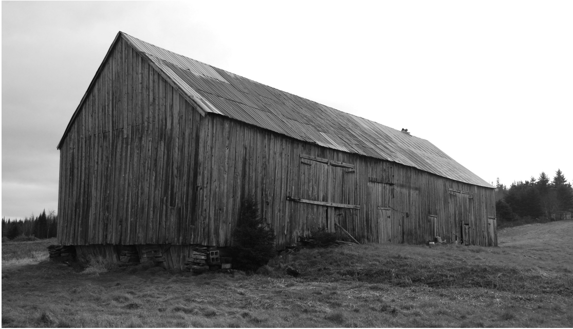
Figure 51. View of Cumminger barn in full double English form, showing the grade of the land. For a desirable siting, land around the barn was probably excavated to ensure a level yard in front of the double doors. Photo by author.
