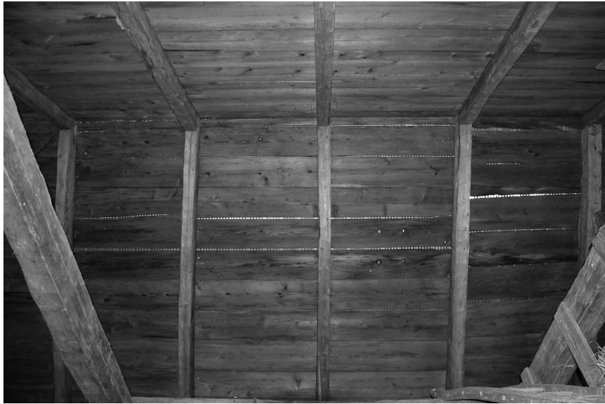
Figure 35. Evenly spaced common rafters in the Cruickshank barn. Note there are no supportive purlins. Photo by author.
