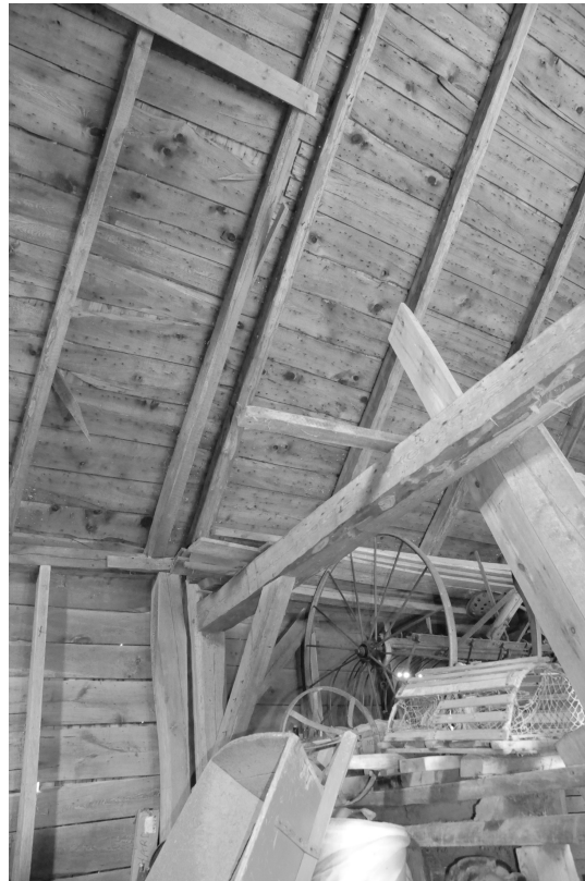
Figure 84. Like the much earlier Cumminger barn, extension was facilitated in the third and final phase of building in the James Fisher barn, Fisher's Mills, by erecting a partial bent next to a complete bent. Clearly, builders of this barn's final extension were conservative in some strategies (facilitating extension) while progressive in others (dimensional studs). Observe that the extension framing is more structurally sound than in the Cumminger barn, as there is minimal separation between the old post and the new. Photo by author.
