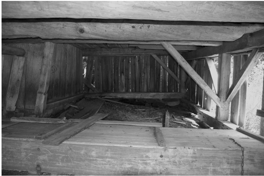
Figure 48. Cellar of Cruickshank barn. Note the bracing coming from the posts. Left is the enclosed sunken hay mow. Photo by author.
