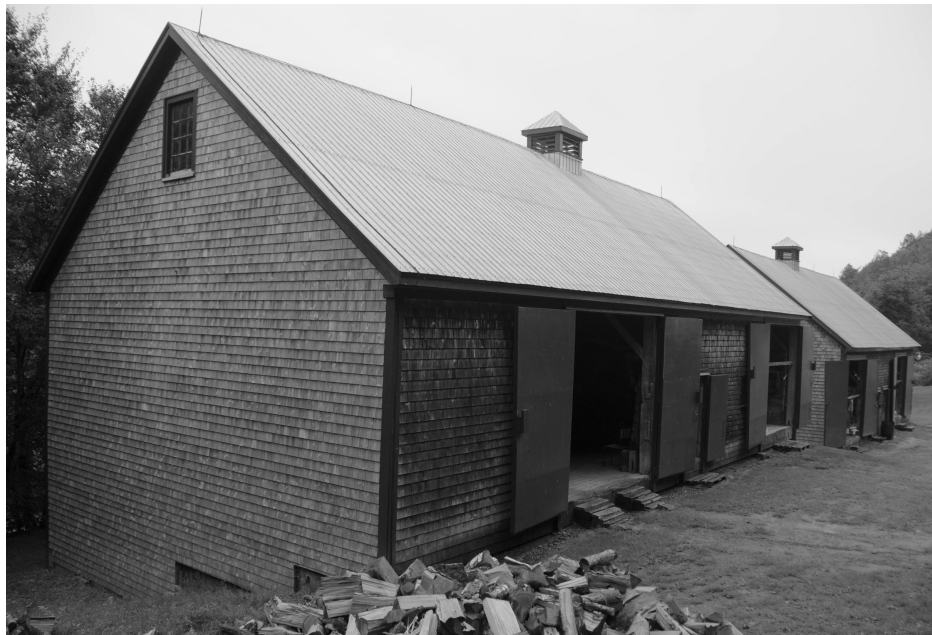
Figure 74. The lower Tom & George Ross barn, Waternish, running NW-SE, 60x30 ft. The barn was built as five bays probably around 1903, when the brothers jointly inherited their father's farm and also built a duplex farmhouse. The lower barn was intended as a sister structure of the upper barn. While the exterior look, dimensions, and interior plan is similar to the upper barn, the framing bent assembly differs. Plan by author and Gerald Pocius. Drawn by author.
