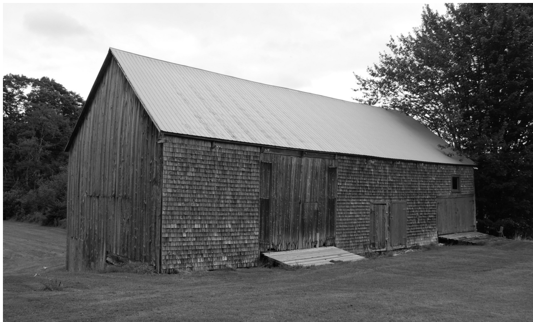
Figure 71. Hattie barn, Hattie Rd., Glenelg. The height of the ESE end bay door is lower than the other floor door, and has a window, indicating that it was primarily used for wagon/equipment storage. Cecil Hattie confirmed that this door, as well as the window above, were a later modification to the structure. Photo by author.
