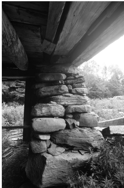
Figure 86. Stone pier (or potentially part of a full wall) supporting both the original English barn sill and the extension sill of the Cruickshank barn. Photo by author.
