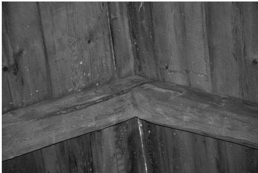
Figure 36. Rafter join in Cruickshank barn. Note there is no ridge pole or board. Photo by author.
