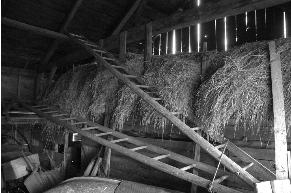
Figure 22. Scaffolding above the stabling bay provided additional loose hay storage and insulation for the animals below. The entry to the passageway for feeding is to the left. Cruickshank barn, Lower Caledonia. Photo by author.
