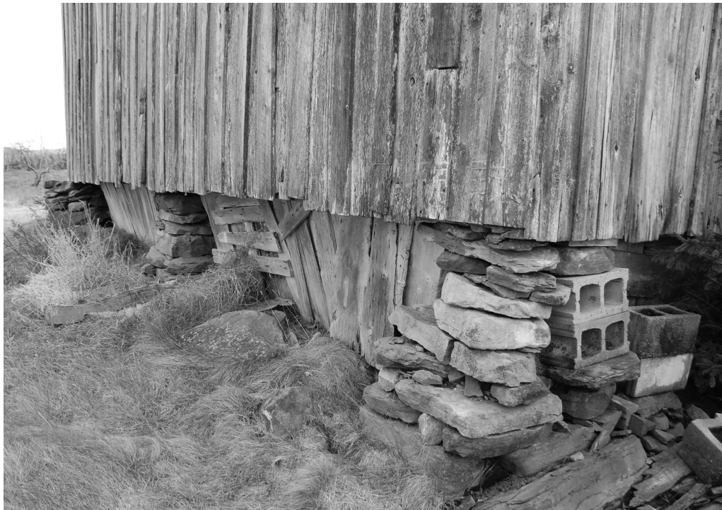
Figure 50. NE gable end of Cumminger barn, Aspen. Three fieldstone piers as well as the vertical board enclosure for the sunken hay mow are visible.
