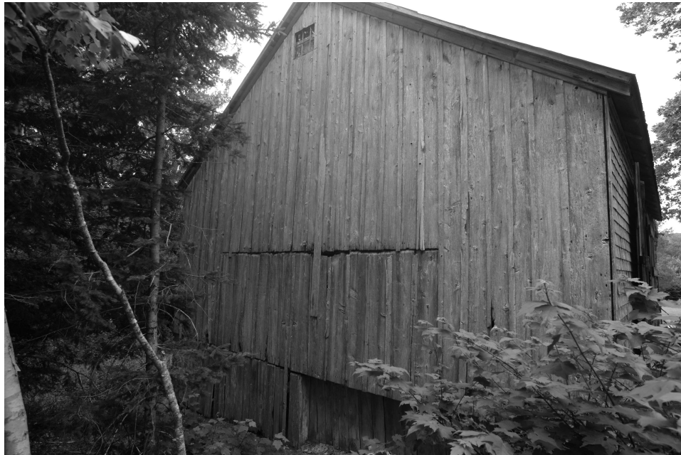
Figure 40. NE gable end wall of the Cruickshank English barn. Original vertical sheathing is visible on the gable end. The battens, as well as the small window in the gable peak, are a later addition. No battens are present in the SW gable end wall (this is the original end of the barn, which the first bent of the extension was raised up against). Note how the barn is on a grade, and that the haymow is sunken below floor level, and protected with vertical boards. Photo by author.
