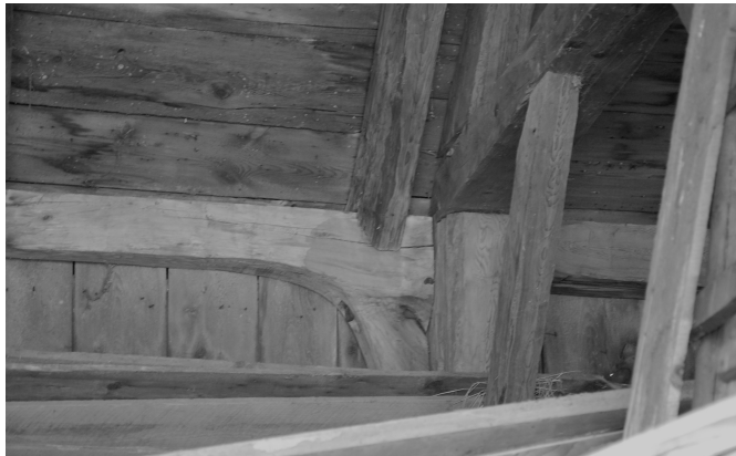
Figure 89. Samuel Archibald barn, Glenelg. The final extension to this barn is facilitated by fashioning the end of the new wall plate as a knee. The knee is bolted to the post of the last bent of the old form. The rafter is seated on the plate as usual (left). The brace on the opposing side of the bay, by the double doors (right). Photos by author.
