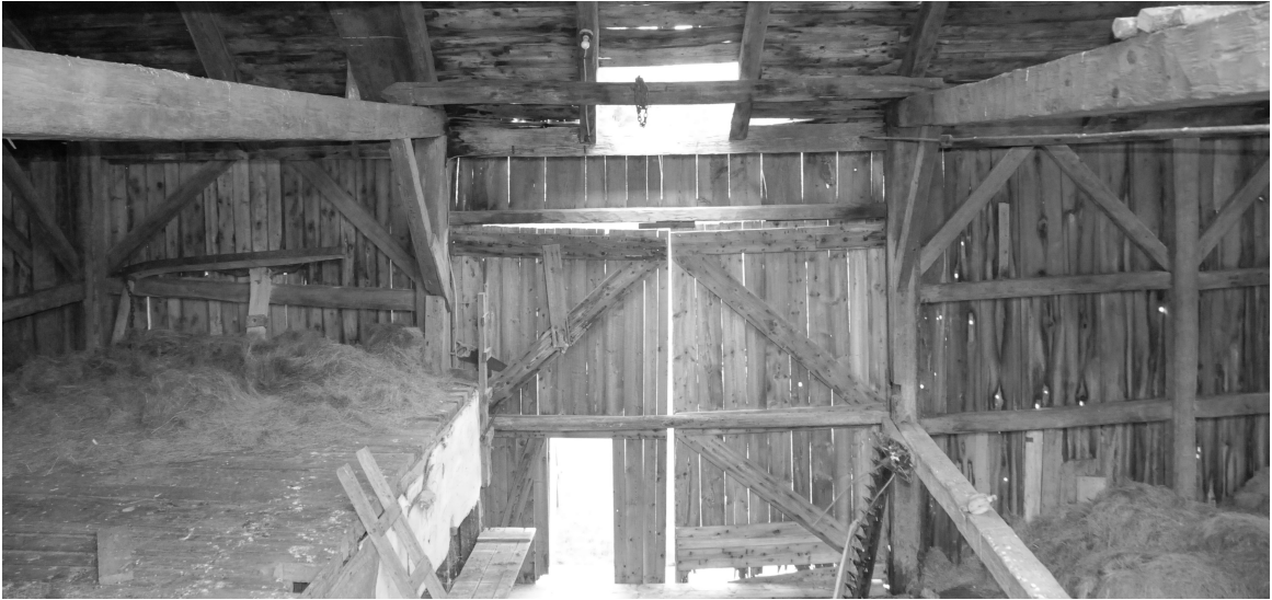
Figure 27. Threshing floor bay of the Cumminger English barn. The log roll with chain for butchering is visible above the double doors, and spans the tie beams.
