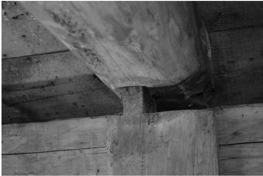
Figure 30. Tenon of a post wiggling out of the mortise of the corresponding tie beam in the James Fisher barn, Fisher's Mills. Photo by author.
