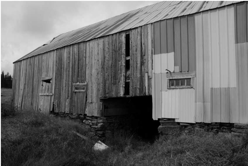
Figure 65. Entrance to manure cellar on the SE lateral wall of the Cumminger barn. The dry stone underpinnings of the barn are visible. Photo by author.
