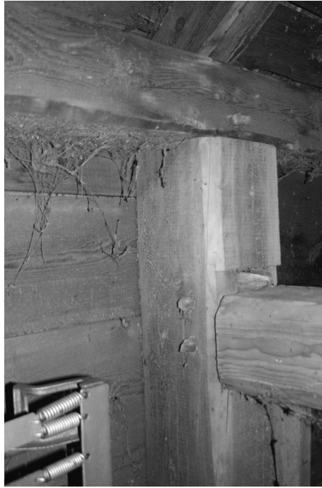
Figure 94. Phase II bent assembly in the Cruickshank barn, East River St. Mary's. The marks of a vertical or reciprocal saw are visible on this post. All major posts in the barn are dimensional, measuring exactly 8 in. x 8 in. Photo by author.
