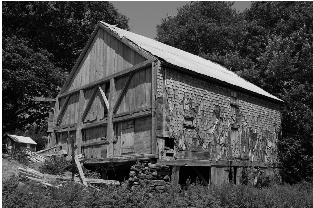
Figure 46. Rear view of Cruickshank barn, Caledonia. Note how the barn is built against the bank to create a cellar level. A large stone pier supports the S corner of the barn. The vertical boards of the original Phase I English barn are visible now that the Phase II mid-century extension is demolished. The exposed Type Ia bent assembly visible against the old vertical boards is all that remains standing of the Phase II extension. Note also the small door in the rear wall for circulation of air to the threshing floor.
