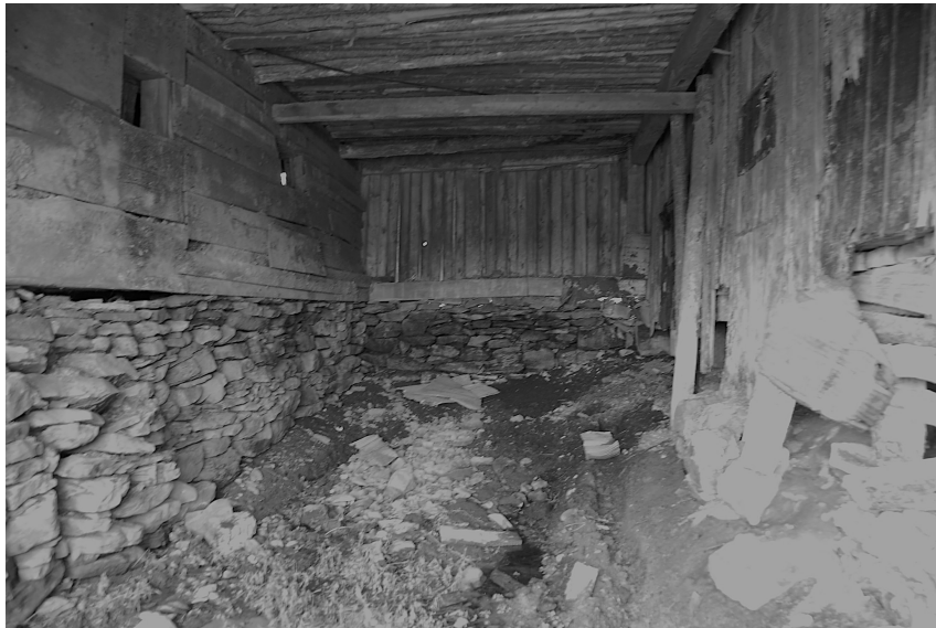
Figure 64. Interior of manure cellar, Cumminger barn. The spruce pole flooring of the loft level hay platform is visible, as are the hatches on both sides of the cellar used to shovel out the cow dung from the byre. Photo by author.
