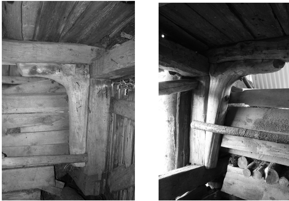
Figure 91. Knee bracing in the cellar level of the John Henry Jordan barn, Newtown. Photo by author.
