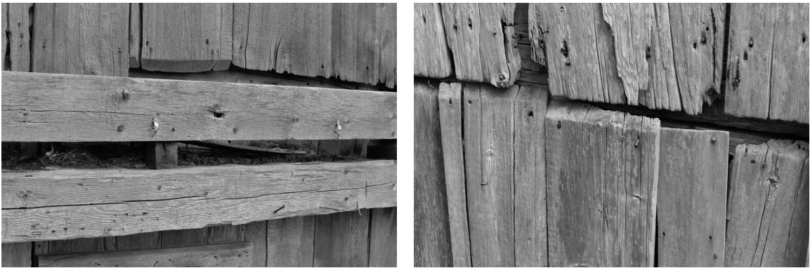
Figure 41. Beveled board edges of the Cruickshank English barn sheathing. NE gable end (left). SW gable end (right). Photo by author.
