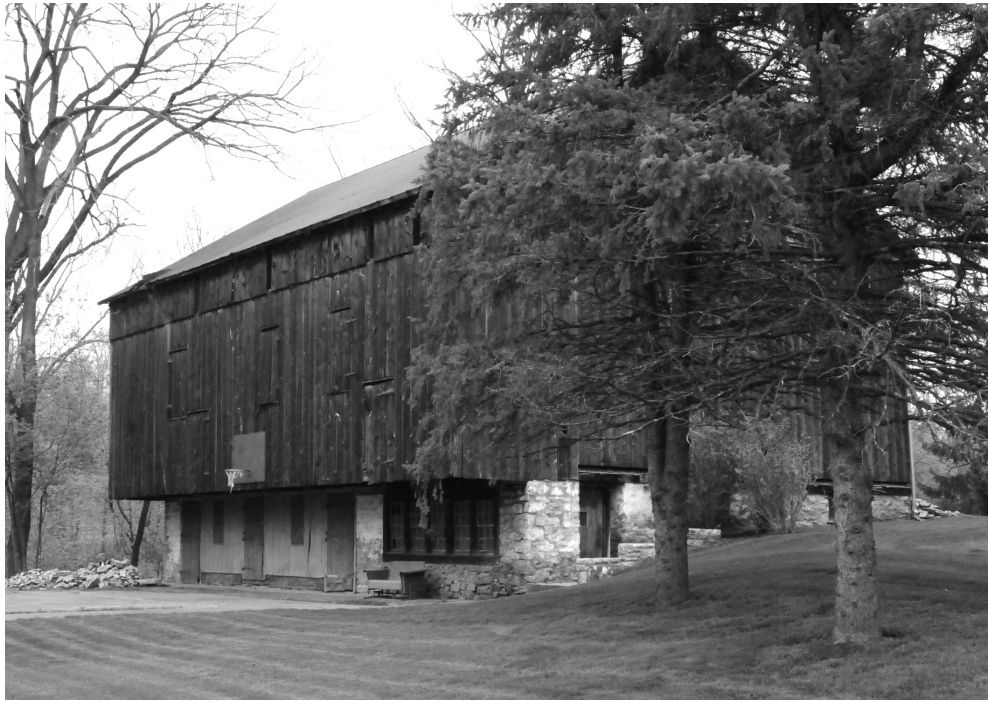
Figure 59. Bank barn with forebay extension and masonry cellar stabling below, near Neff's Mill covered bridge on the Pequea Creek, Penn Grant Rd., Lancaster County, Pennsylvania. Photo by author.
