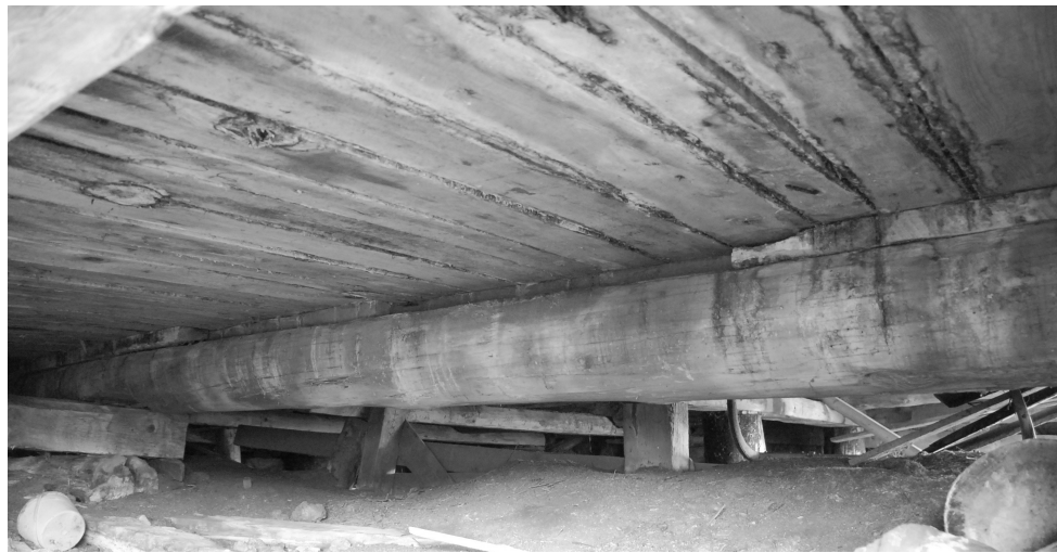
Figure 43. View from under the Cumminger barn, showing a large, in-the-round floor joist. Photo by author.
