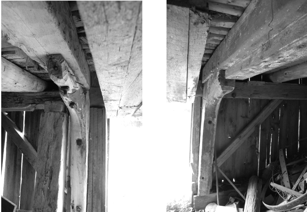
Figure 90. Knee bracing in the cellar level of the Hattie barn, Glenelg. The braces are positioned on either side of the door to the cellar. Photo by author.
