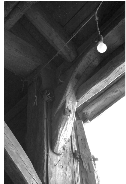
Figure 89. Samuel Archibald barn, Glenelg. The final extension to this barn is facilitated by fashioning the end of the new wall plate as a knee. The knee is bolted to the post of the last bent of the old form. The rafter is seated on the plate as usual (left). The brace on the opposing side of the bay, by the double doors (right). Photos by author.
