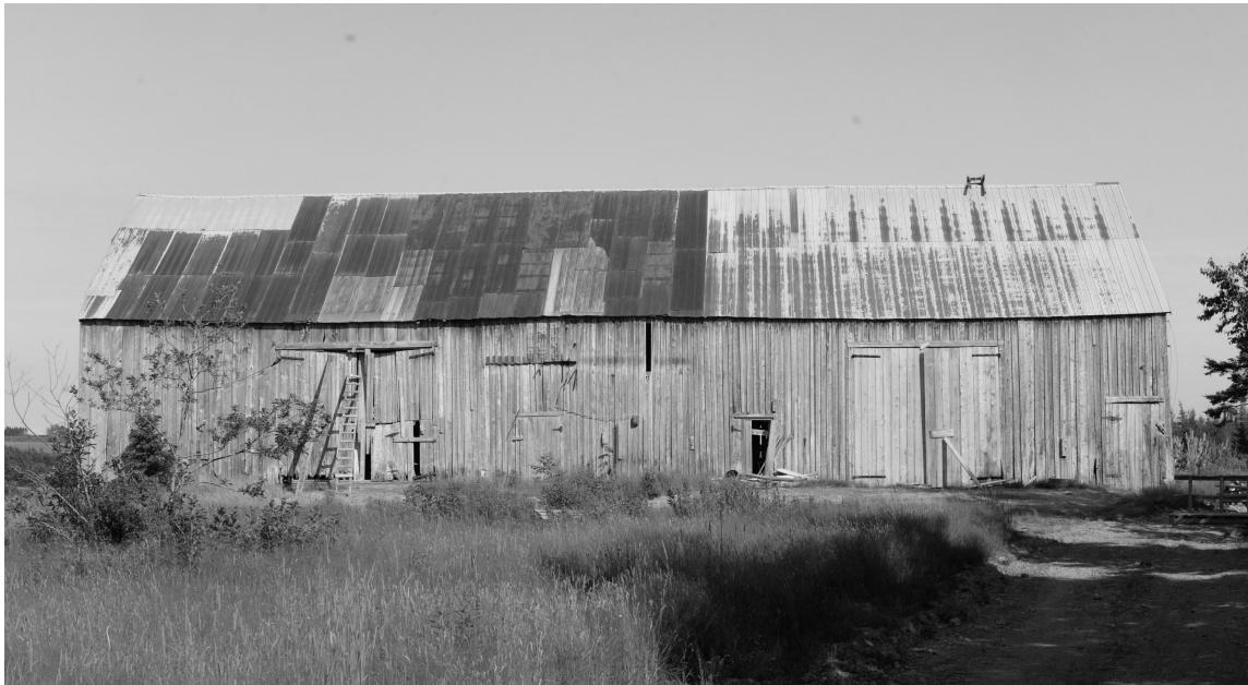
Figure 63. Samuel Cumminger's eight bay extended barn. The large space of wall at the dead center of the barn, between the two small stable doors, is where the manure cellar is positioned. The faint scars of a former mid-twentieth century milk house is also visible. Photo by author.
