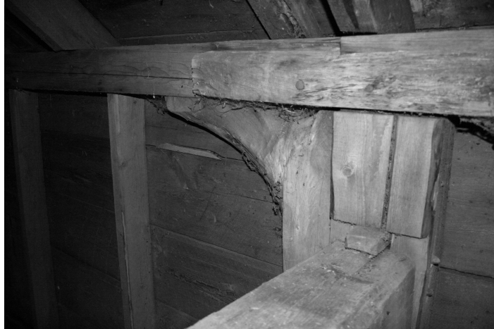
Figure 88. William G. Cruickshank barn, East River St. Mary's. A grown knee brace bolted to the post facilitates the joining of an additional bay to the original two-bay asymmetrical barn, built circa 1889 (see the following chapter for further analysis of this barn). Photo by author.
