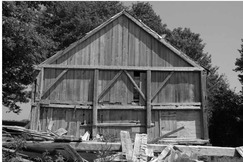
Figure 85. Cruickshank barn, Lower Caledonia. The exterior vertical sheathing of the English barn is shown, as well as the two doors used to access the extension from the barn’s interior. The bent of the extension is positioned directly against the sheathing. Photo by author.
