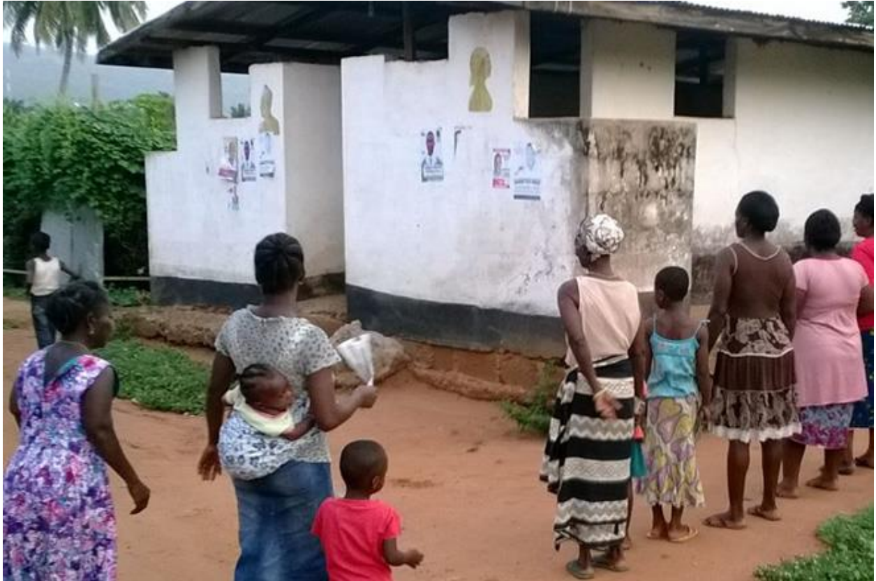
Figure 2: A toilet facility in Ghana.
