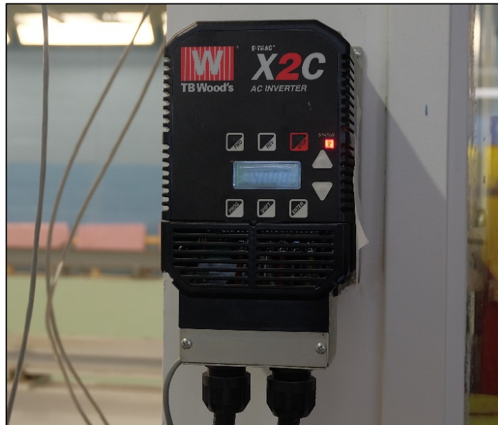
Figure 3.2: TB Wood AC Inverter.
