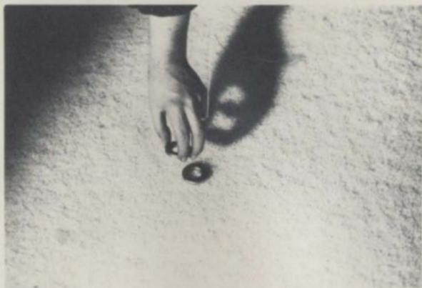
Fig. 5. Load-deflection test of model ice sheet.
