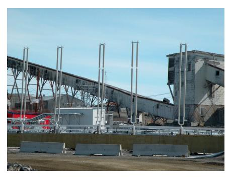
FIG. 11.3: Thermosyphon test plot, Giant Mine Remediation Project. Photo by John Sandlos.
