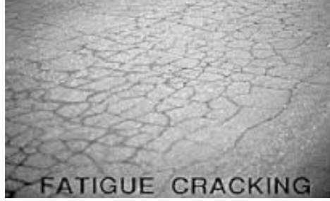
Figure 1.3: Damage in the wheel track as a result of fatigue failure, in a further phase fatigue cracks [3].
