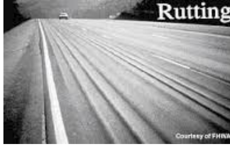
Figure 1.4: Rutting under highest tonnage and high temperatures [3].
