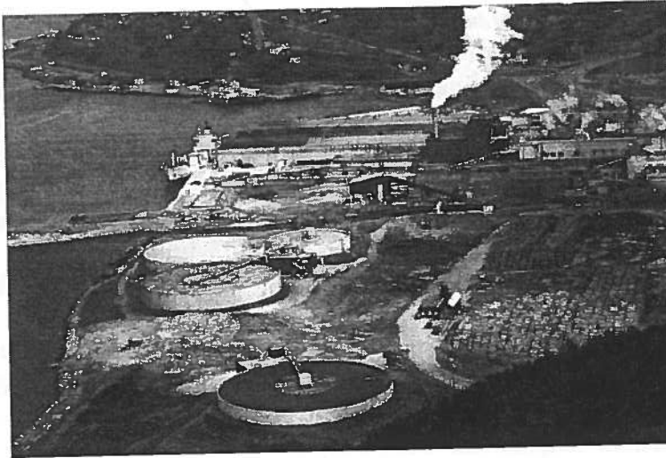
Figure 3. Oblique View of the Mill (Dept. of Environment and Conservation, n.d.)
