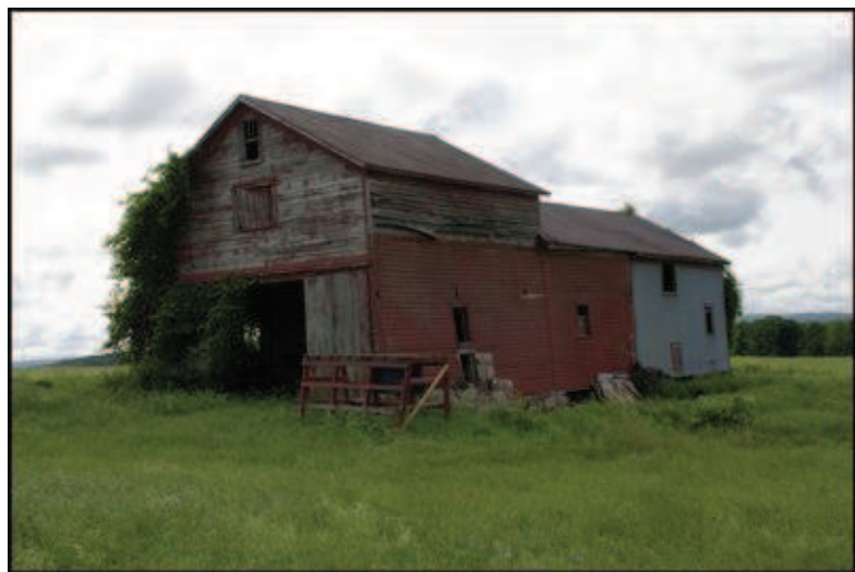
FIGURE 4.21 THE PATTERSON HOP HOUSE, TOWN OF SPRINGFIELD.
