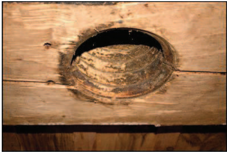
FIGURE 3.14 SCREW BEAM HOLE, CHASE HOP HOUSE, TOWN OF MIDDLEFIELD.
