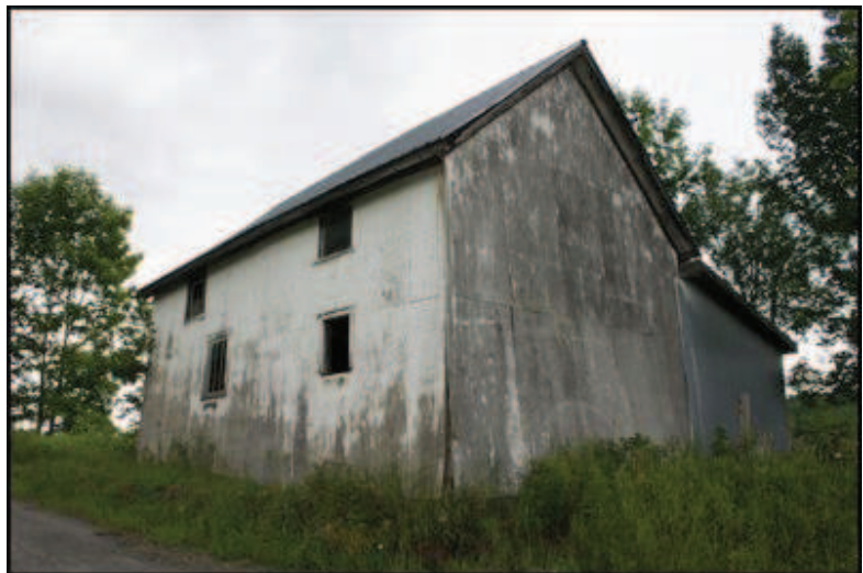
FIGURE 4.47 THE THERING HOP HOUSE, TOWN OF HARTWICK.
