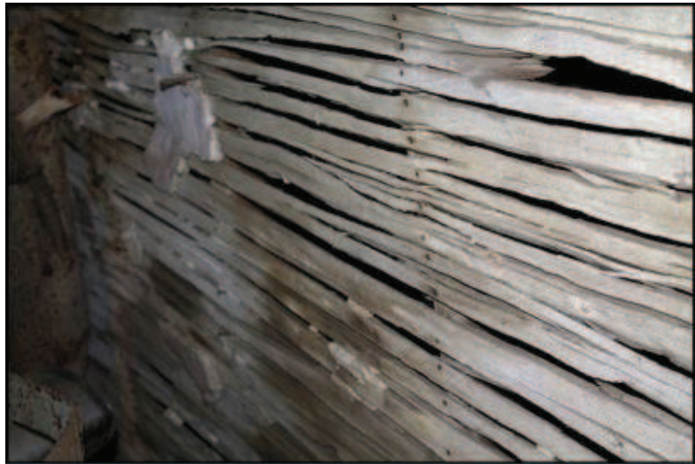
FIGURE 3.7 PLASTER AND LATH, H. SMITH HOP HOUSE, TOWN OF SPRINGFIELD.
