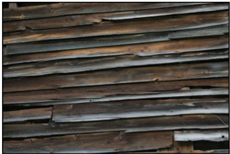
FIGURE 3.21 CLAPBOARD SIDING, H. SMITH HOP HOUSE, TOWN OF SPRINGFIELD.
