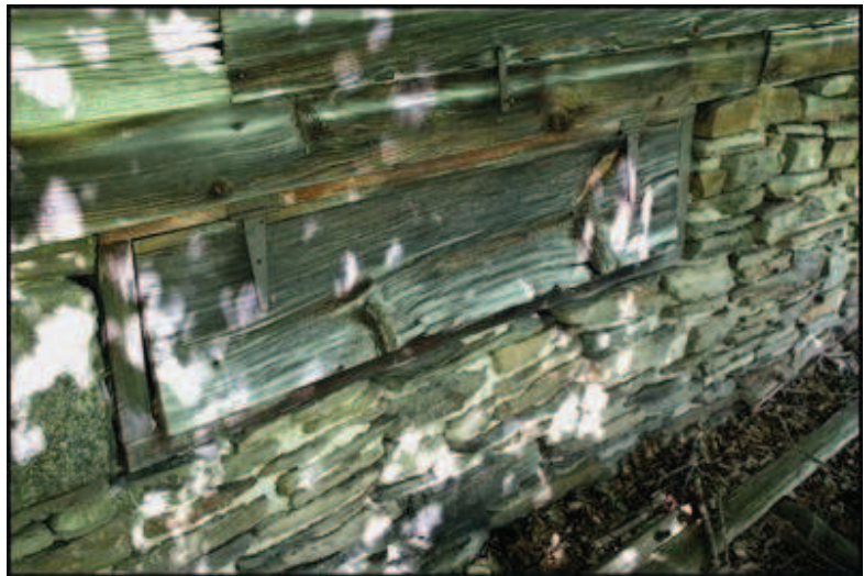
FIGURE 3.3 KILN VENT, LEE HOP HOUSE, TOWN OF OTSEGO.
