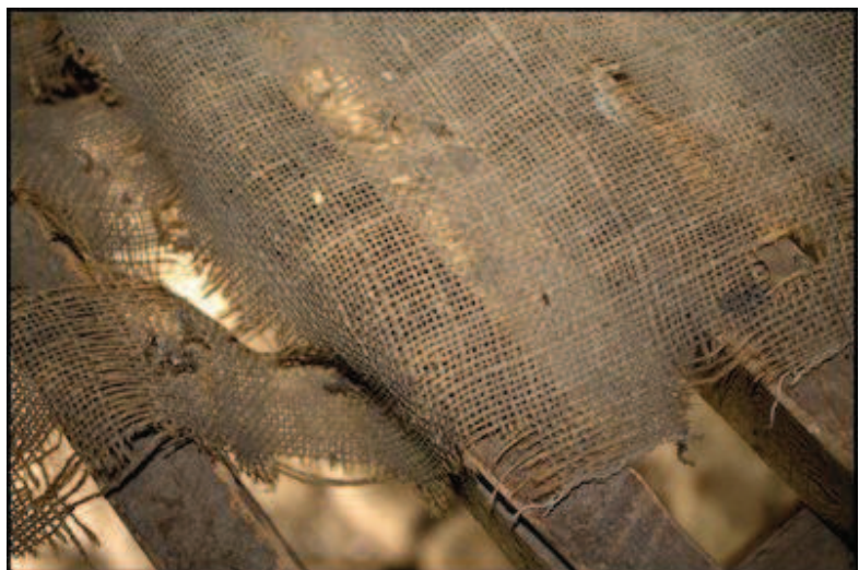
FIGURE 3.6 DRYING SLATS, SONDERGAARD HOP HOUSE, TOWN OF DECATUR.
