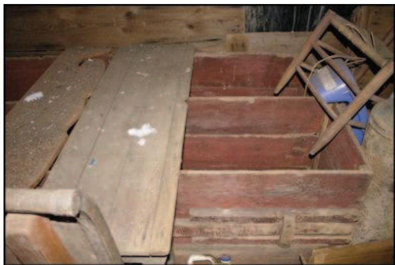
FIGURE 5.1 HOP BOX. H. SMITH HOP HOUSE. TOWN OF SPRINGFIELD.
