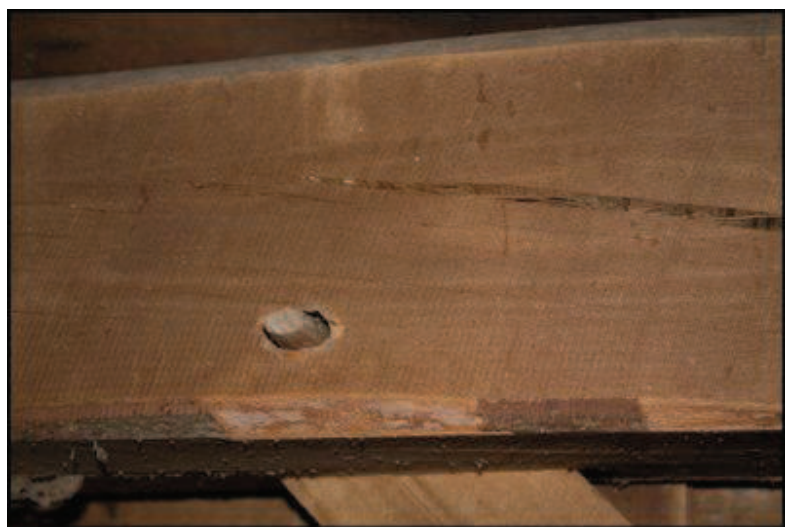
FIGURE 3.16 CIRCULAR SAW MARKS, SEAMON HOP HOUSE, TOWN OF EXETER.
