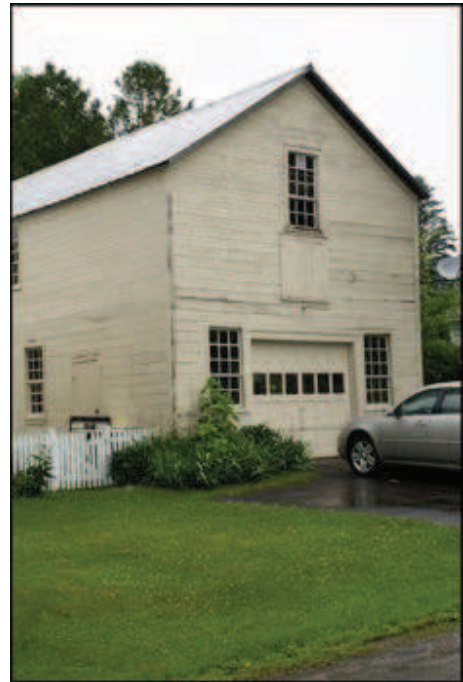
FIGURE 4.54 THE EVERS HOP HOUSE. TOWN OF ROSEBOOM.
