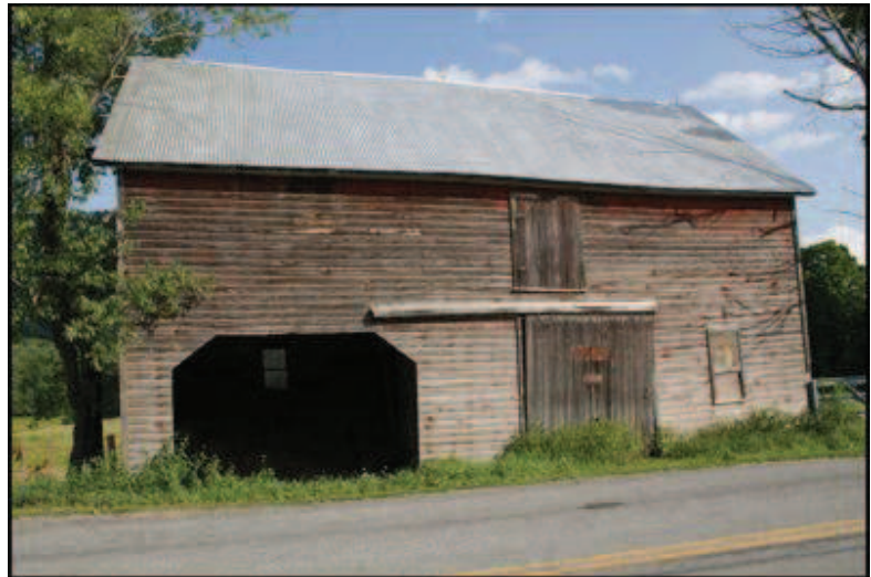
FIGURE 4.62 THE SONDERGAARD HOP HOUSE, TOWN OF DECATUR.
