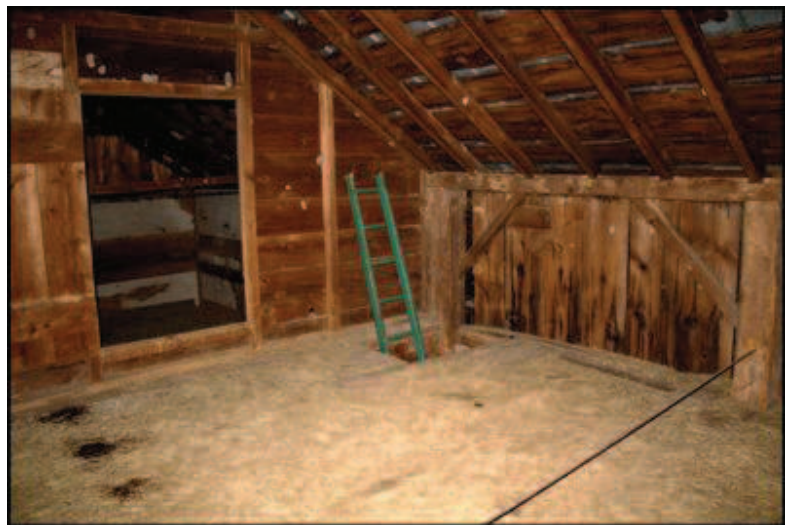
FIGURE 3.10 STORAGE ROOM, KNAPP HOP HOUSE, TOWN OF OTSEGO.
