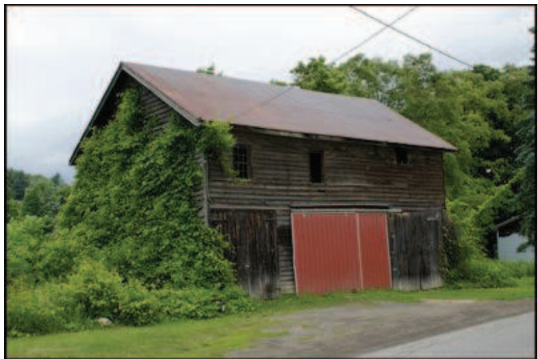
FIGURE 4.29 THE A. SMITH HOP HOUSE, SALT SPRINGVILLE, TOWN OF CHERRY VALLEY.
