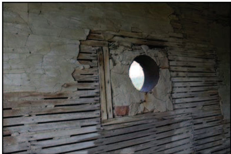
FIGURE 4.63 BRICK AROUND PIPE EXIT, SONDERGAARD HOP HOUSE, TOWN OF DECATUR.
