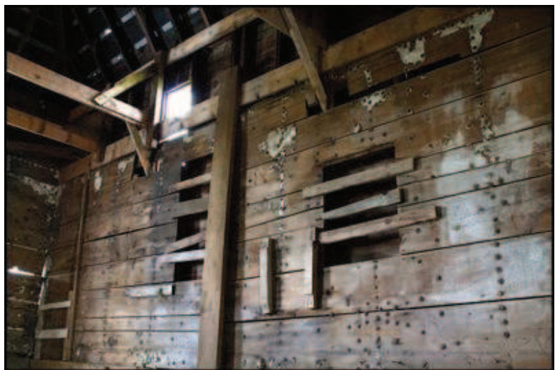
FIGURE 3.9 ASBESTOS LINED KILN, KARKER HOP HOUSE, SCHOHARIE COUNTY.
