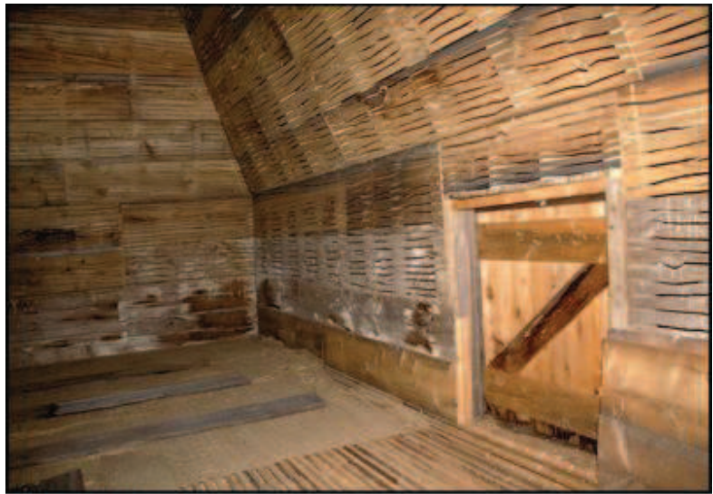
FIGURE 3.8 LATH CEILING, BEARDSLEE HOP HOUSE, TOWN OF PITTSFIELD.
