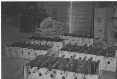
Fig. 4.3 Preparation for steel reinforcement
