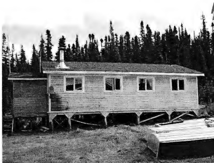
The outside of the guides' cabin. Photo by L. Nippard, Summer 2010.
