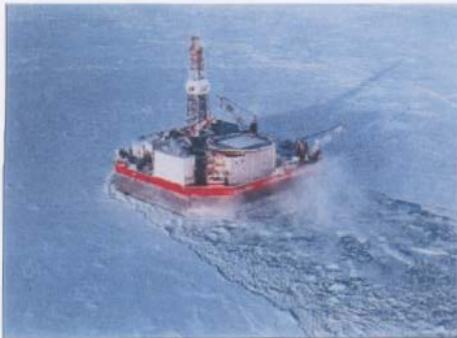
Figure 8-4: The Molikpaq in the Beaufort Sea. Illustrating how a stationary structure being impacted by a large floe is comparable to an indenter test.
