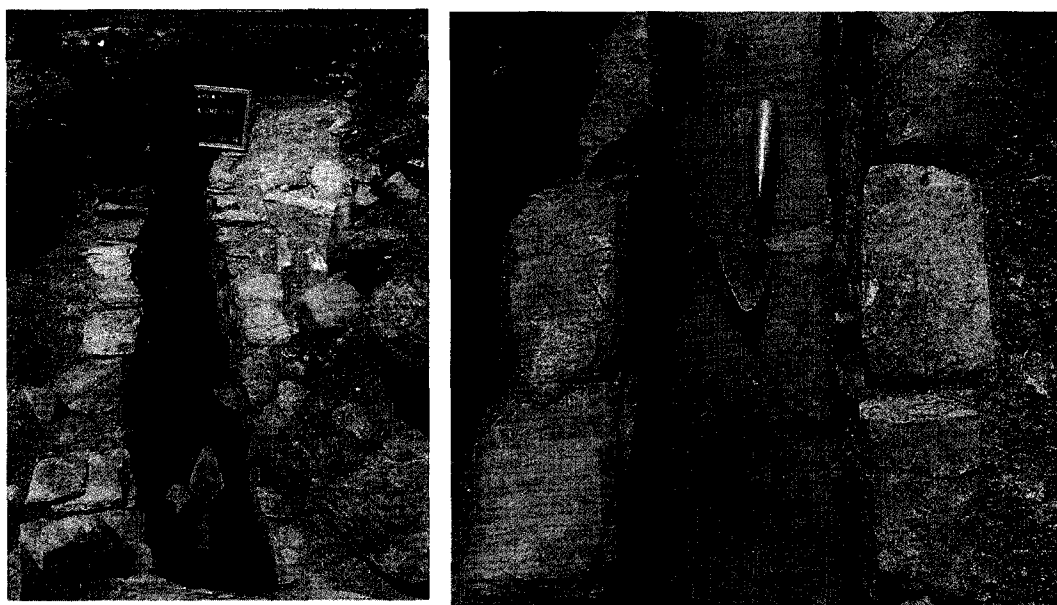
Figure 13. (left) Slate drain associated with the brewhouse/bakery; (right) detail of drain showing the use of roof slate to level the walls.
