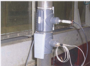
Figure 4.3: Pressure and Temperature Sensors with Clamp-on Saddles
