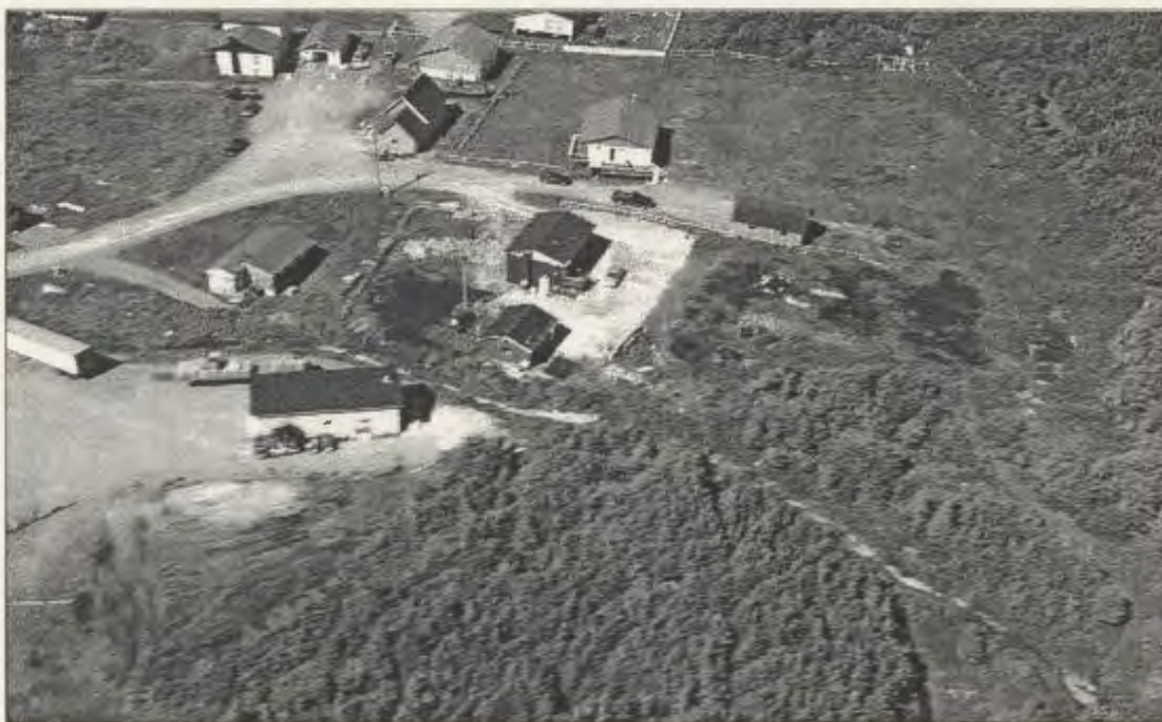
Figure 2.3 – Aerial photo of the Gould property where most excavation was conducted.
