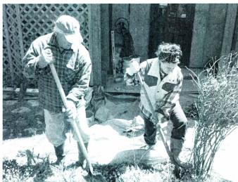
Figure 19. Len and Michelle in perfect unison, digging holes for structural posts, c. early summer 2009. Photograph taken by Marilyn Hollett.
