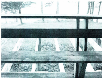
Figure 20. Original seat and railing still intact with new structural layout started, c. 2009.
