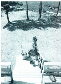
Figure 16. View of new deck stairway from balcony above, c. 2009.
