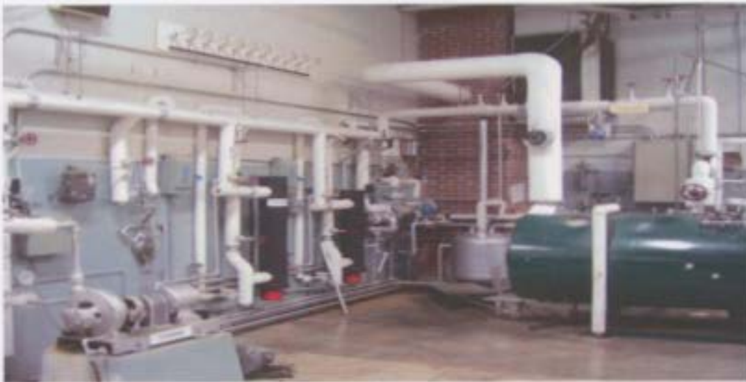
Figure 17 The picture of steam power unit
