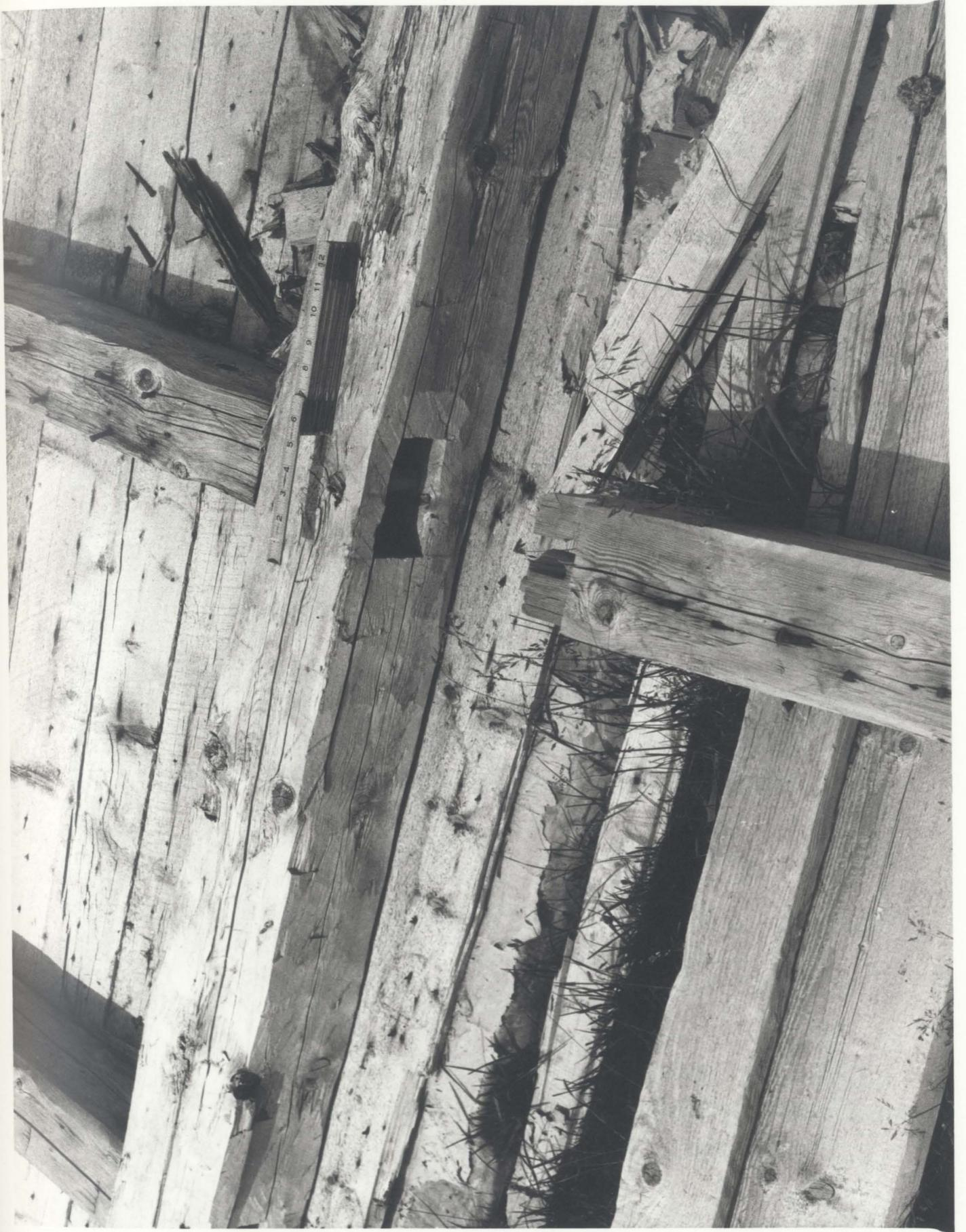
Figure 79 Construction details showing typical framing members in a wall bent at Norman McIsaacs's house, Upper Ferry. This bent consists of 8 upright, hand-hewed studs morticed into a top and bottom plate with two diagonal corner braces supporting the frame. The exterior sheathing consists of saw-milled boards laid diagonally to provide more strength to the frame.
